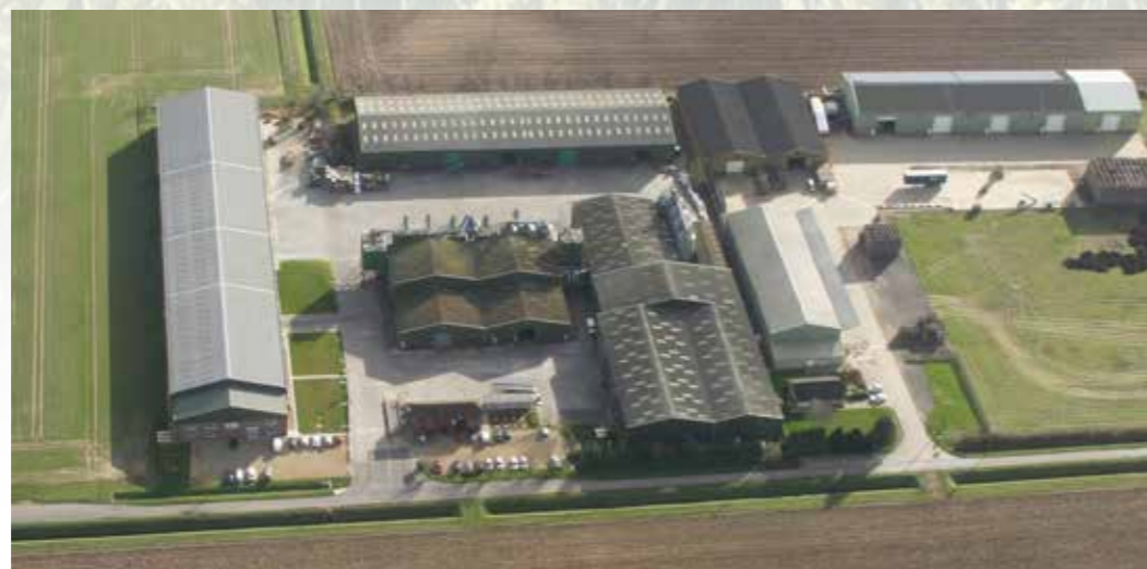
ADM's seed processing plant at Long Sutton
